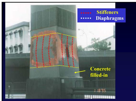
**DAMAGED STEEL BRIDGE PIER IN THE HYOGO-KEN NANBU EARTHQUAKE, 1995**
