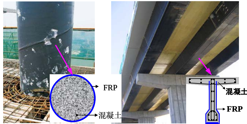
FRP-RC composite column/beam
