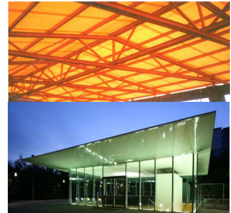
FRP light roof
