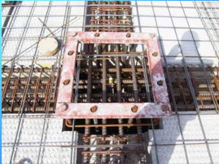
A device for the alignment of column longitudinal reinforcement
